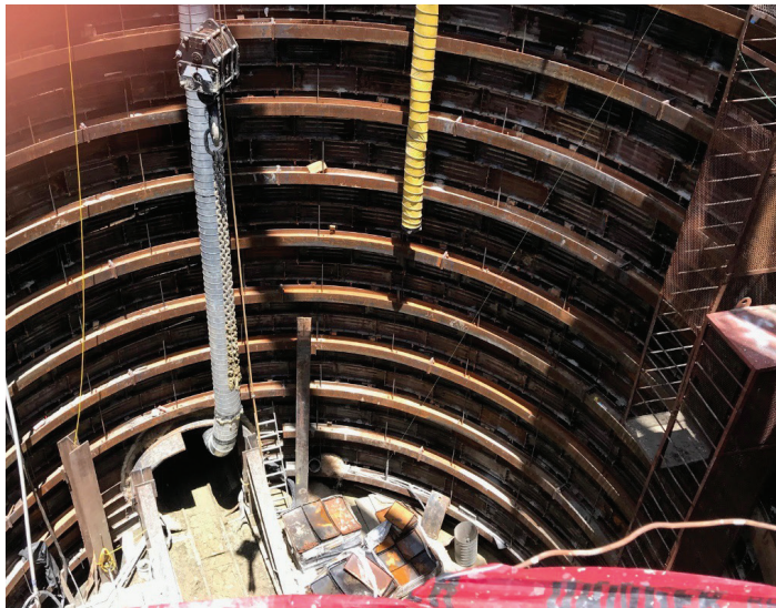
The water line construction required a pit 100-ft in diameter, and 75-ft deep. The electrically-powered excavation machine is positioned inside the tunnel pictured at the bottom of the photograph.
