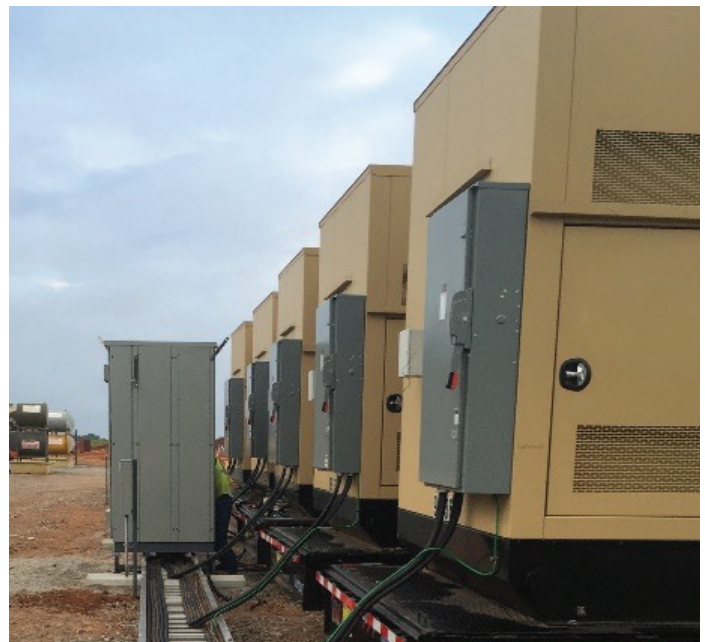
Baseline 3.5 MW natural gas generator microgrid in operation for Oklahoma gas and electric utility.
